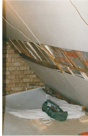
Timber framed walls for extension and sloping roof of loft conversion insulated with Celotex boards
