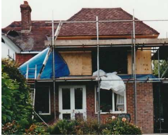
Timber framed walls for extension and sloping roof of loft conversion insulated with Celotex boards
