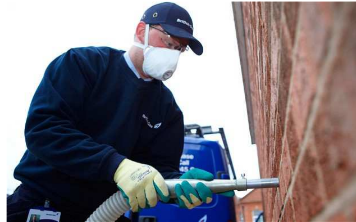
Cavity wall insulation
