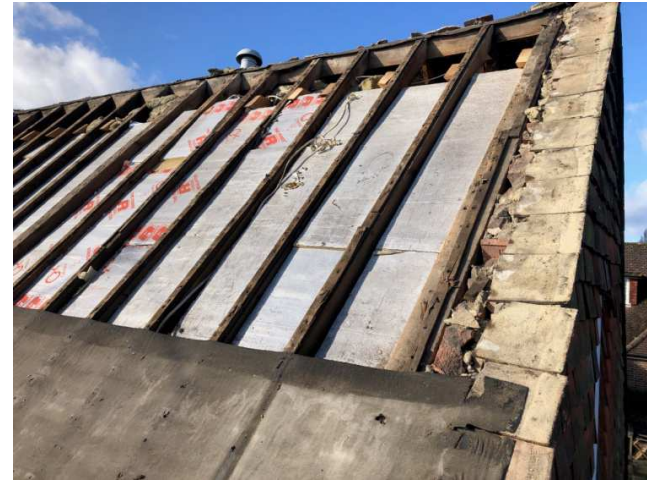
Timber framed walls for extension and sloping roof of loft conversion insulated with Celotex boards
